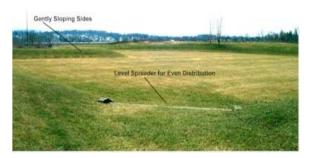
An Infiltration Basin is a shallow impoundment that stores and infiltrates runoff over a level, uncompacted, (preferably undisturbed area) with relatively permeable soils.
