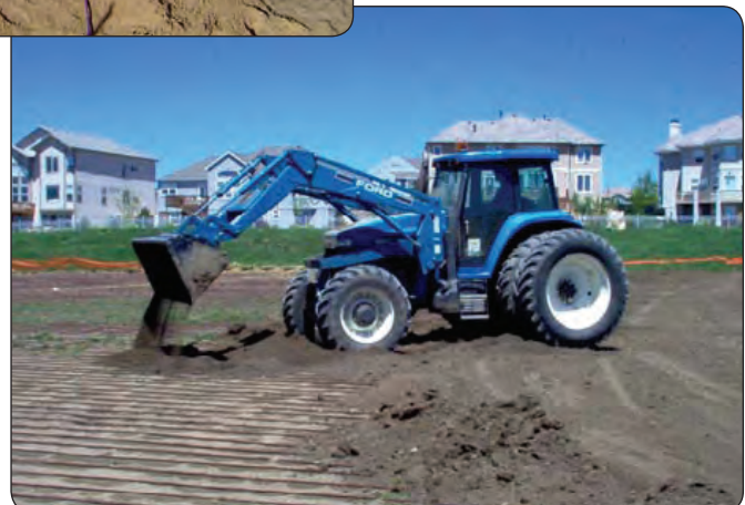
Figure 20 - Mechanized Equipment May be used to spread soil over the top in larger systems. It is important to evenly spread the soil moving with the tubing direction to keep the laterals from shifting.
