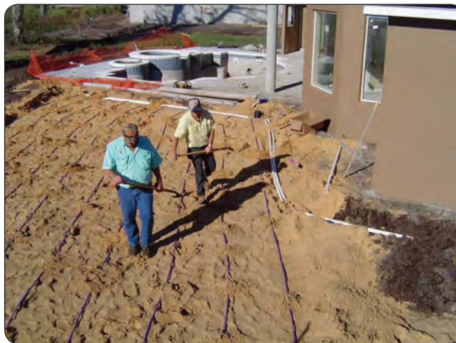
Figure 19 - "Drip and Fill" Technique.
